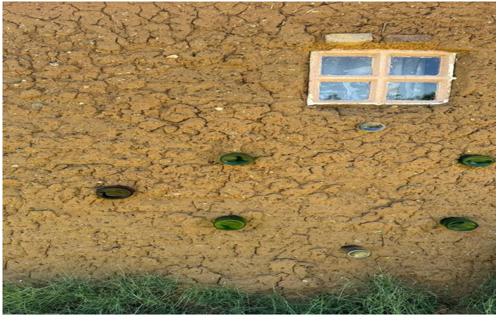
Figure 3: Earthen wall construction at Meraka cultural village
