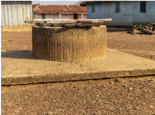
Fig 5.5 A well constructed by Prophet Oppong (for the Akontanim community)
